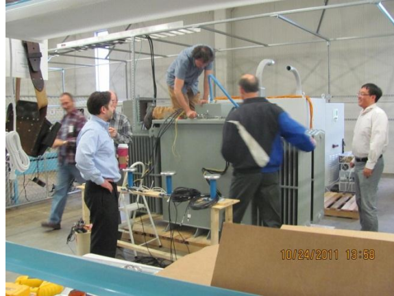
High-Voltage Enclosure (800 VAC \leftrightarrow 50 kVDC) Includes xformer in oil
