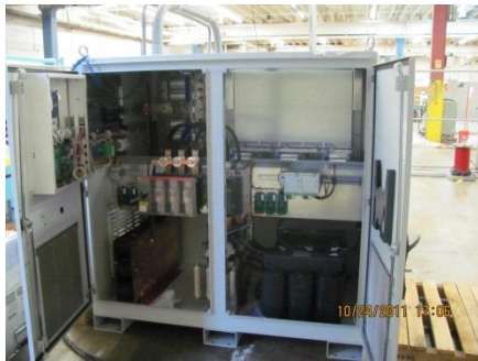
Low-Voltage Enclosure (480 VAC \leftrightarrow 6-8 kHz 800 VAC)
