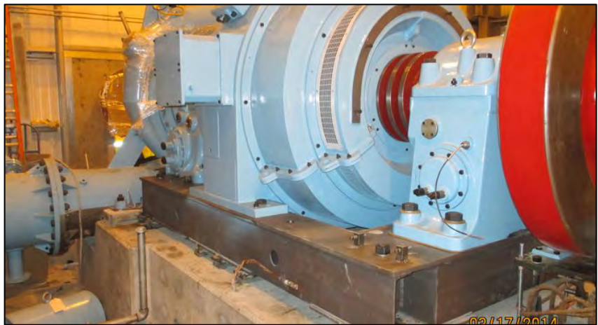
Whitman Lake Hydroelectric Project Photos: Dawson Construction
