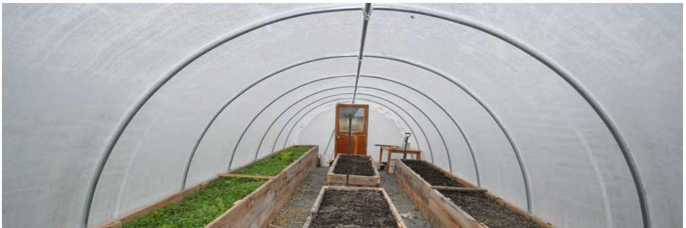
Newly constructed high tunnel in Haines.
