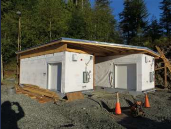
Thorne Bay biomass under construction
