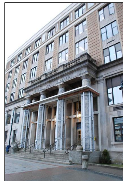
Braces on Marble Columns, State Capitol
