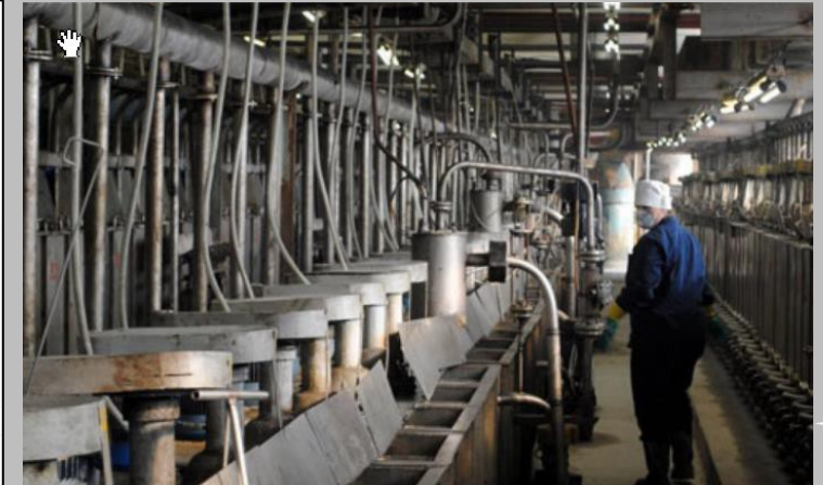
An operator monitoring the mixer-settler levels at the NPM Silmet rare-earth separation plant, located in Sillamäe, Estonia. Photo: Joel Tozer
