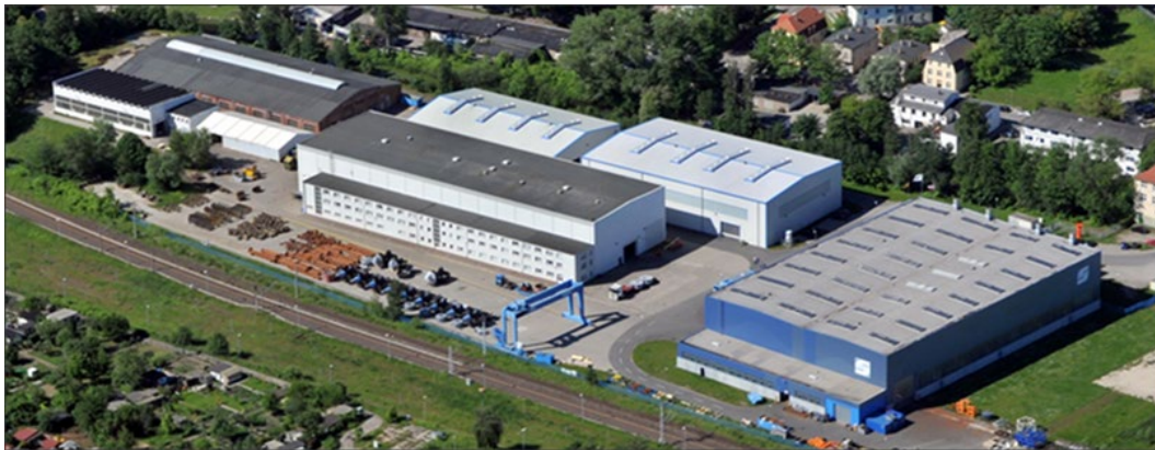
Schottel Factory-Wismar Germany
