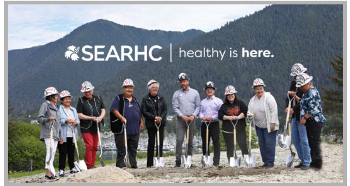
Mt. Edgecumbe Medical Center Groundbreaking June 2022
